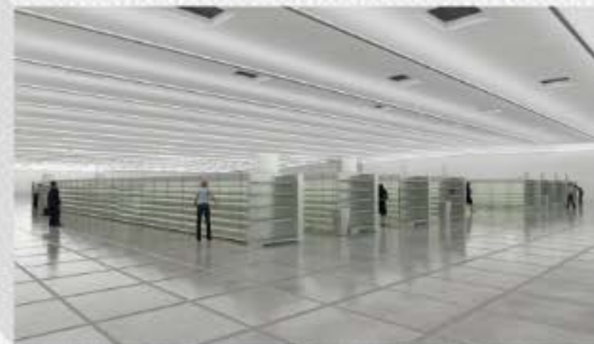
Ceiling Lighting at 100% Shelf Lighting at 0.25W/ft
